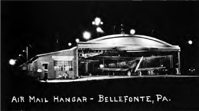
Above: Air mail hangar lit by floodlights.
